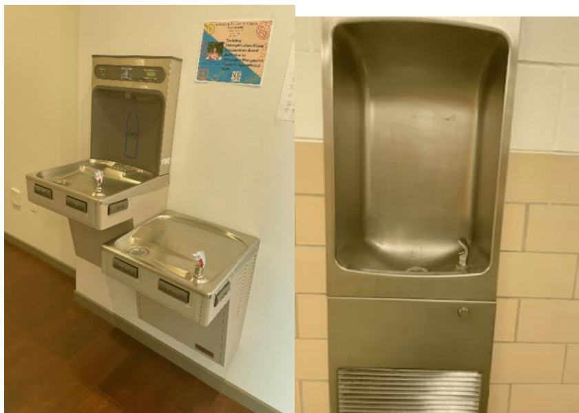
Figure 21. Hydration stations and water fountains in the Nettie Stevens Science and Innovation Center and Wilson Hall, respectively. Notice the design of the hydration station in the Science and Innovative Center, with the station having reusable water bottles in mind. (Caitlyn Murphy)
